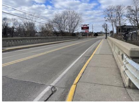
Bridge Over Clinton River
